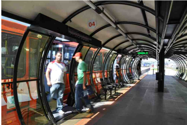
Transfer station shelter, Curitiba. Brazil
