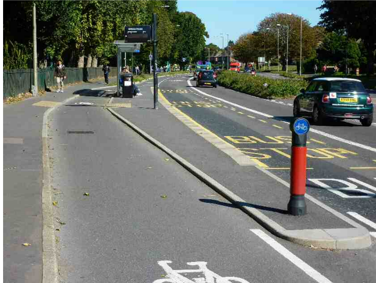
[Bus stop and cycle bypass, Brighton, England. Note use of kerbs to distinguish road space from pedestrian footpath, and gradual path curvature to reduce the inconvenience of horizontal deviation.]
