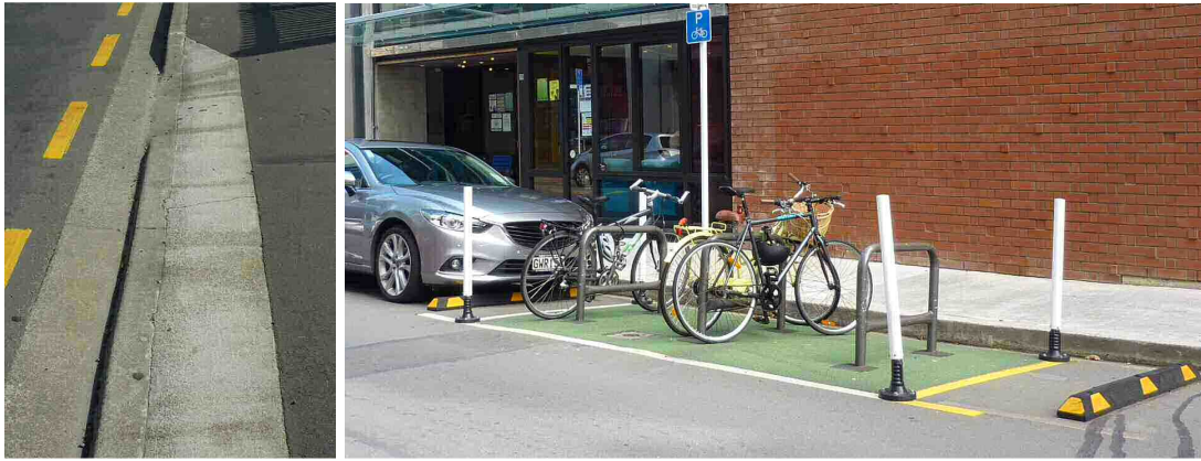
Figures 4 and 5: Dropped lip in driveway, Willis St (nr intersection with Karo Drive); replacing car parks with bike parks, Wigan St
