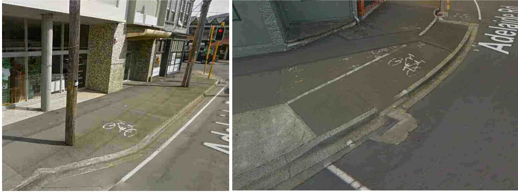
Figure 3: dropped kerb cycling infrastructure, Adelaide Rd
