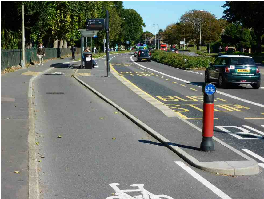
Cycleway and bus stop design, Brighton, England showing levels and kerbing distinguishing road space from pedestrian space, and the gradual curve to the cycleway to accommodate a bus stop island (also note the lack of driveways disrupting the cycleway).
