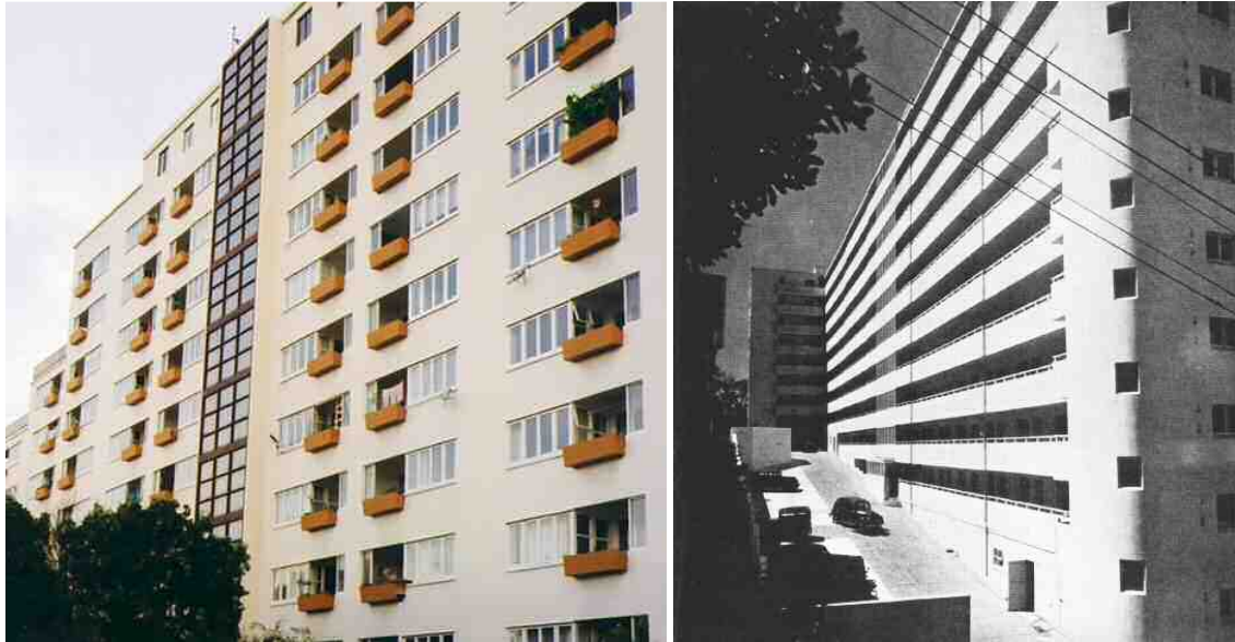
Dixon Street Flats: eastern elevation | western elevation
