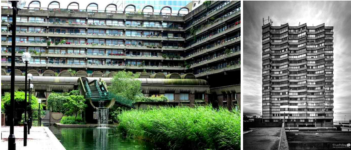
Barbican, London (left) | Arlington Towers, Margate (facade modulated to maximise view and sun) (right).
