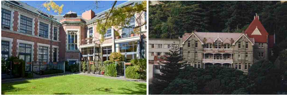
Peterborough apartments, Christchurch (left) | Erskine College, Island Bay, Wellington (right)
