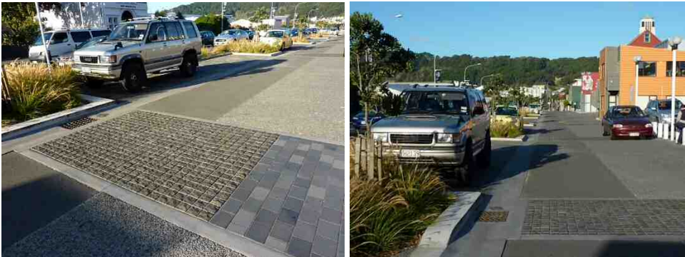
Karo Drive - designed primarily with cars in mind. The rubble strips being an example of this.
