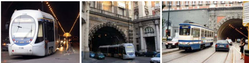
Vittoria tunnel, Naples, Italy.
