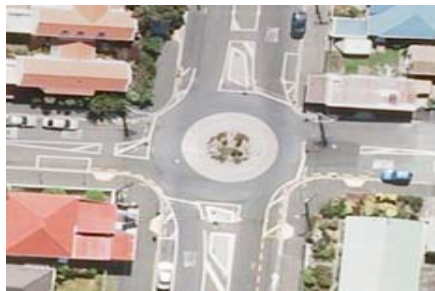
Figure 1: Existing Dee St/Parade intersection with roundabout
