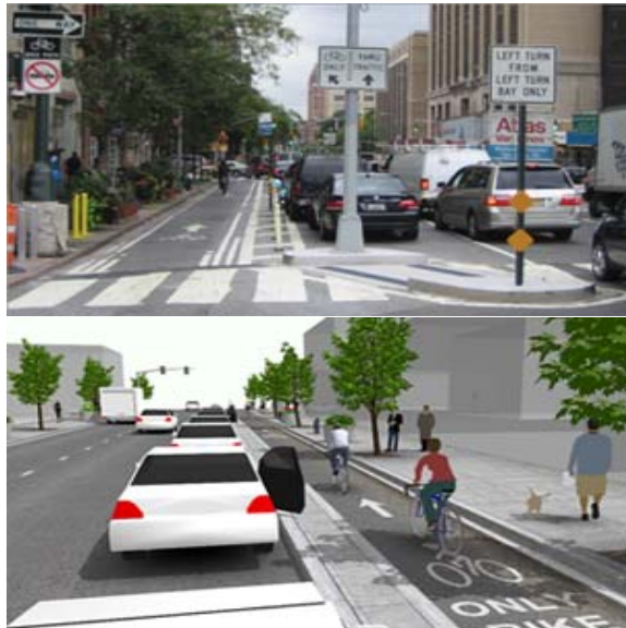
Figure 4: examples of One-way protected Cycle Tracks with Parking from the NACTO Design Guide
