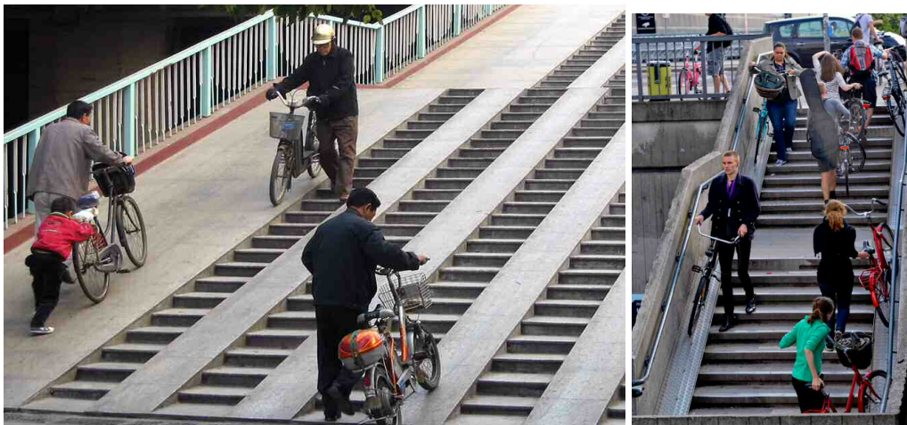
Figures 1 and 2: bike stairway, China; bike gutters, Portland
